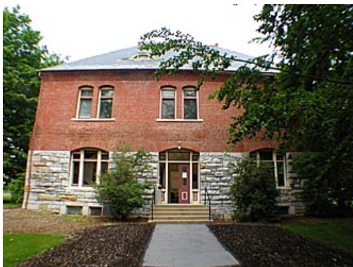
Old Botany Building was completely re-wired as part of the Telecommunications Infrastructure Upgrade Project. Built in 1887, it is the oldest academic building on the University Park campus
